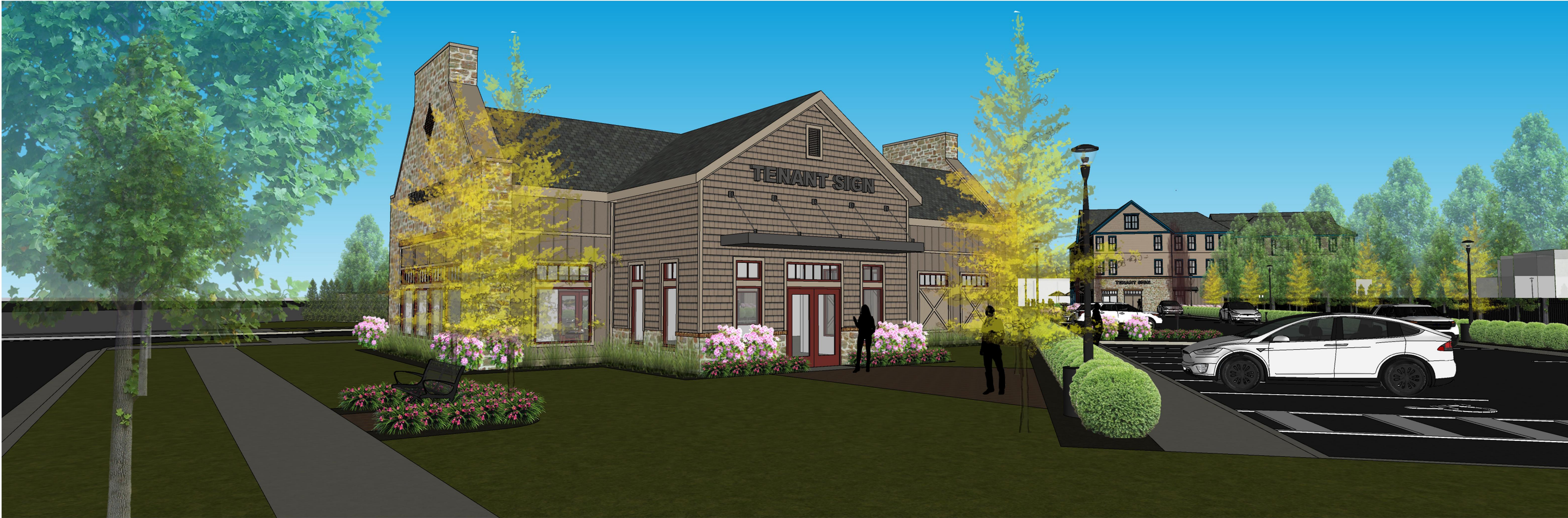
VIEW LOOKING NORTHEAST - BUILDING C
