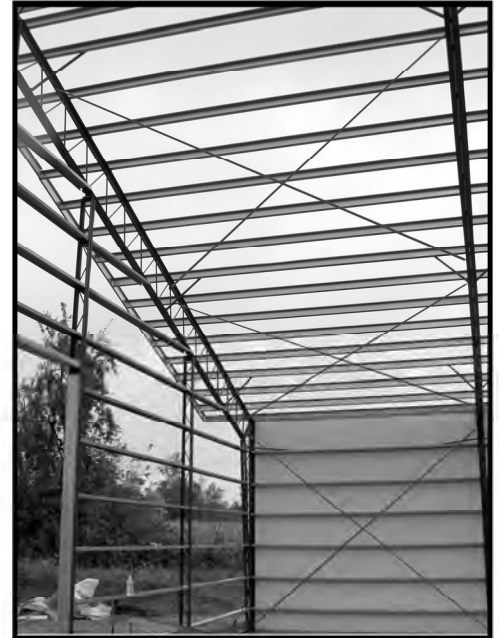
Wind Bay Roof & Wall Cables
