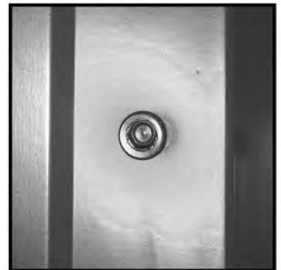
Correct Screw w/washer snug to panel surface.
