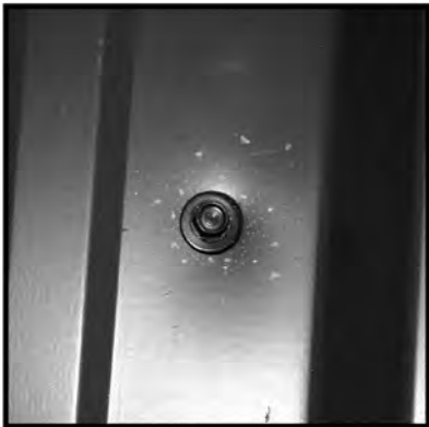
Incorrect Overdrilled screw with steel shavings left on panel
