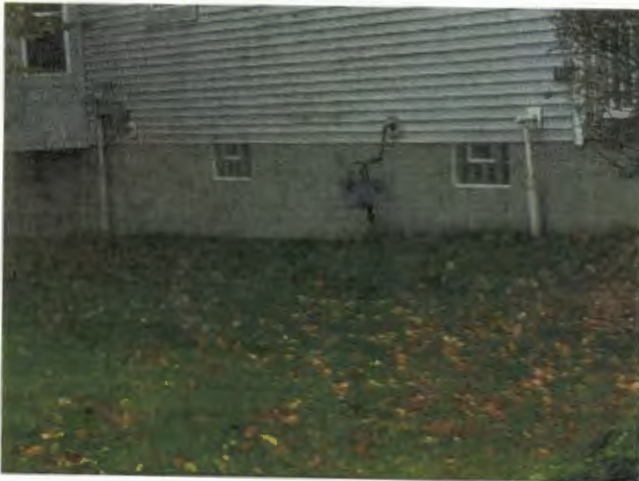
Painted Block Foundation
