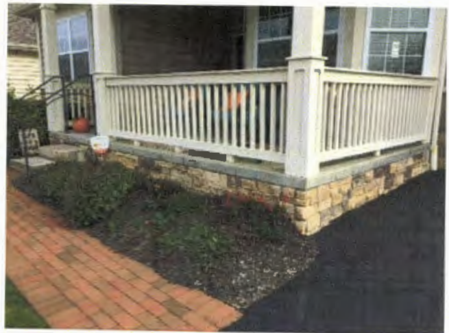
Porch Finished Foundation
