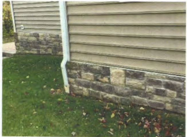
Stone Finished Foundation
