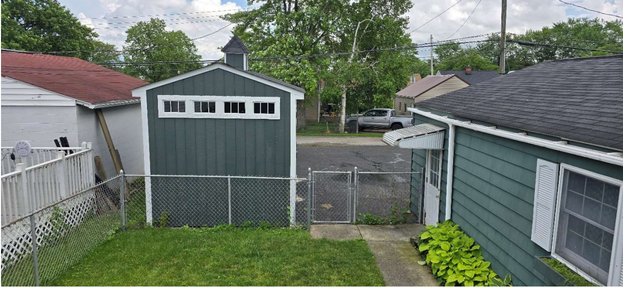
Backyard View NEW SHED
